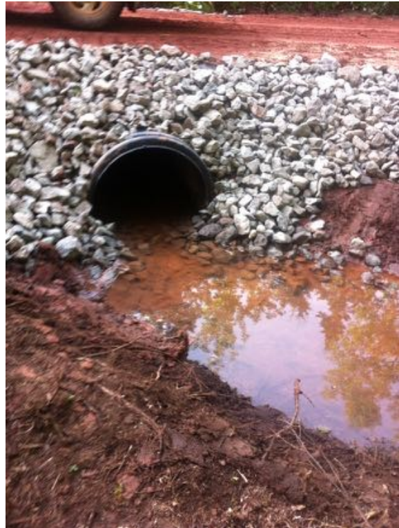
New 3ft Culvert installed.
