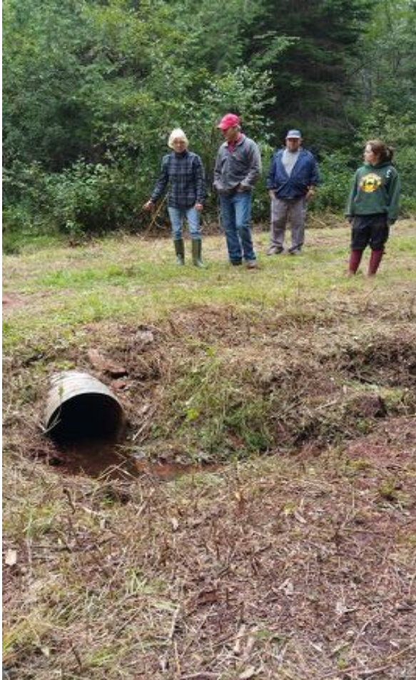
OLD 1.5 FOOT CULVERT
